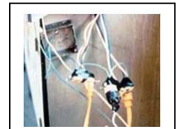
Improper Wiring
