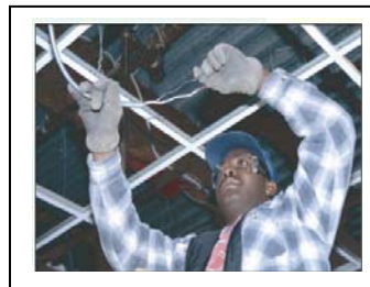
Wear Correct PPE
